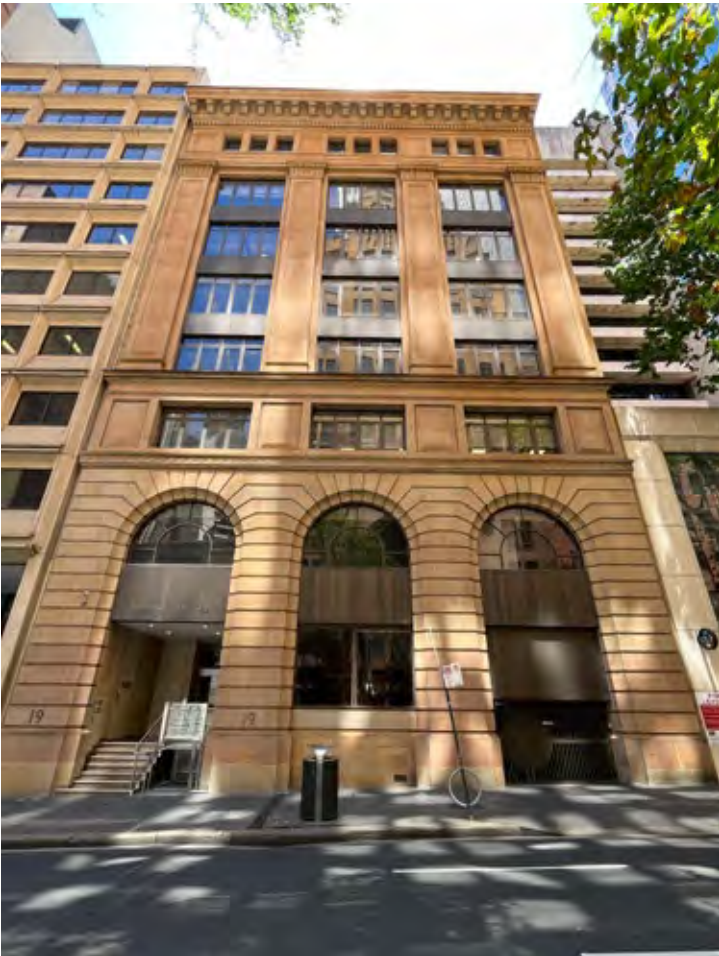
THE PUBLIC TRUSTEE BUILDING (Rofe Chambers) 19-21 O’Connell Street Completed: 1925 Architects: HE Ross and H Ruskin Rowe of Ross & Rowe
