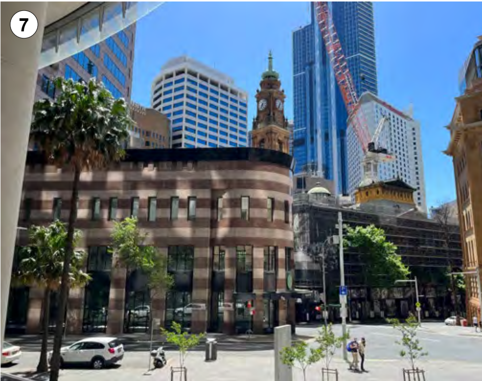
217 View of existing wintergarden building facing north-west, with the Department of Lands Building behind, taken from the steps of 1 Bligh Street (Department of Lands Building currently with scaffold covering the exterior). The existing post-modern wintergarden building design forms an acute point at the northern tip of the site.
