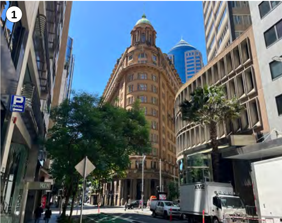
216 The Radisson Hotel (former Wales House) to the corner of Pitt Street and O'Connell Street and Hunter Street as viewed here from Pitt Street facing north. The iconic corner facade with copper dome is a distinct and well known city corner.
